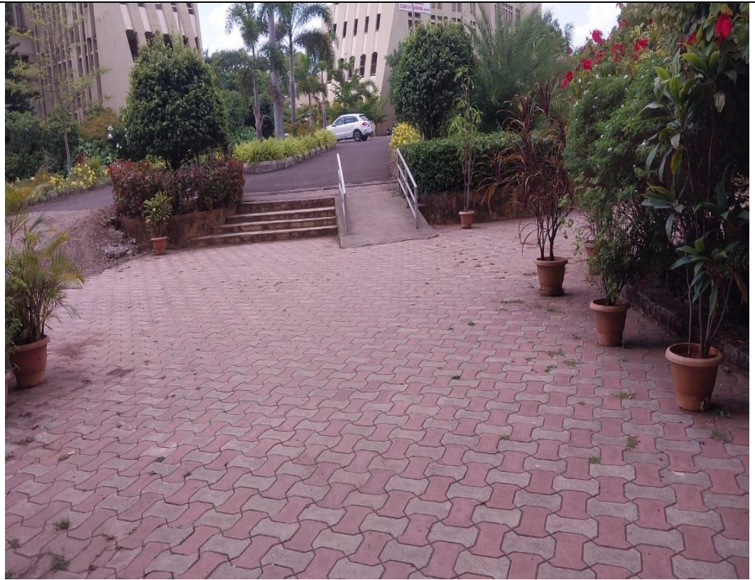
Facilities for disabled
